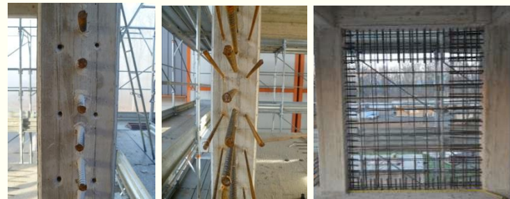
Dowels, starter bars and web reinforcement
