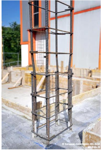
Reinforcement detail for columns
