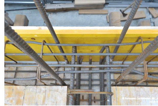
Reinforcement detail for beams
