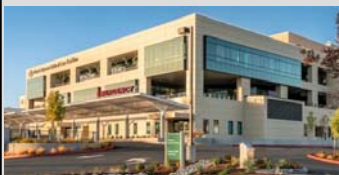
COURTESY: WASHINGTON HOSPITAL ENGINEER: THORNTON TOMASETTI, SAN FRANCISCO
