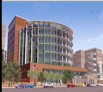
ENGINEER: ARUP, SAN FRANCISCO COURTESY: SAN FRANCISCO DEPARTMENT OF PUBLIC HEALTH
